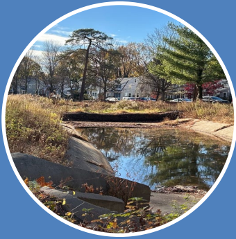
Sediment Detention Basin
